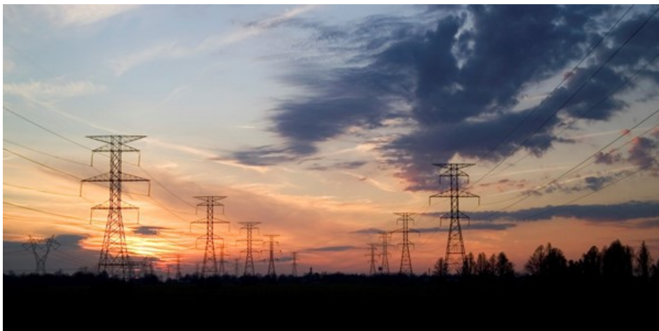
New Madrid Power Plant transmission lines | AECI
